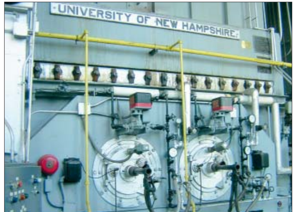
Natural gas and number 6 fuel oil are burned in furnaces at UNH's Central Heating Plant to create steam for heating buildings and hot water for sinks and showers. There are five furnaces in the plant, two using oil, and three that are dual fuel.
