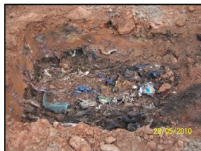
Step 1: Removing soil cover
