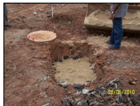
Step 2: Surface regularization
